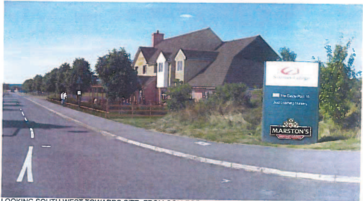
LOOKING SOUTH WEST TOWARDS SITE FROM COLLEGE ENTRANCE OFF EXISTING ROUNDABOUT
